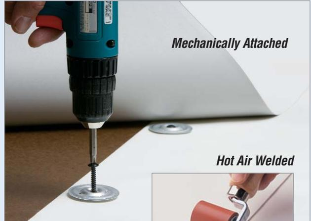
**Flex Thermoplastic Residential Roofing is mechanically attached to the roof. Then the seams are welded with hot air. The seam is as strong as the material it joins.**
